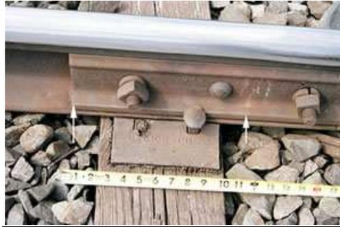
Creep in rails denotes longitudinal movement of rails in the track.
