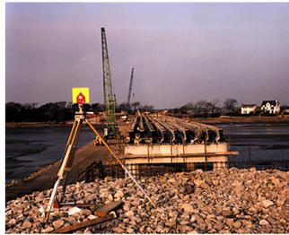
Simply supported concrete beams and slab bridges are now giving way to integral bridges which offer the advantages of less cost and lower maintenance due to the elimination of expansion joints and bearings.
