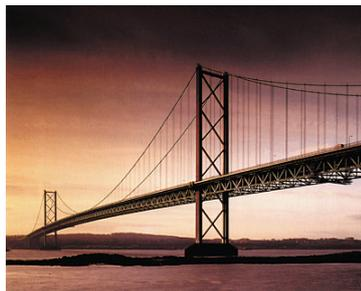
**Stiffened suspension Bridges:-** In stiffened type suspension Bridges moving loads are transferred to the cables through medium of trusses called **stiffening girders**. The stiffening girder assists the cable to become more rigid and prevent change in shape and gradient of roadway platform. It is therefore adopted for heavy traffic.
